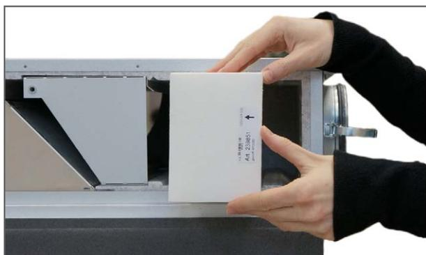
5. The pollen filter is inserted into the marked trail and the door is closed again.
